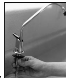
FIGURE 4 - INSTALLING FAUCET
