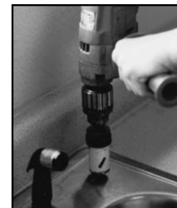
FIGURE 3 - DRILLING 1" HOLE FOR FAUCET
