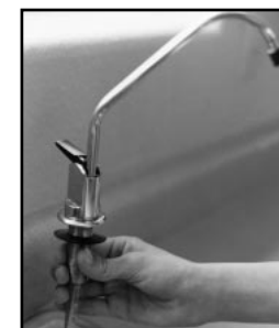
FIGURE 4 - INSTALLATION DU ROBINET
